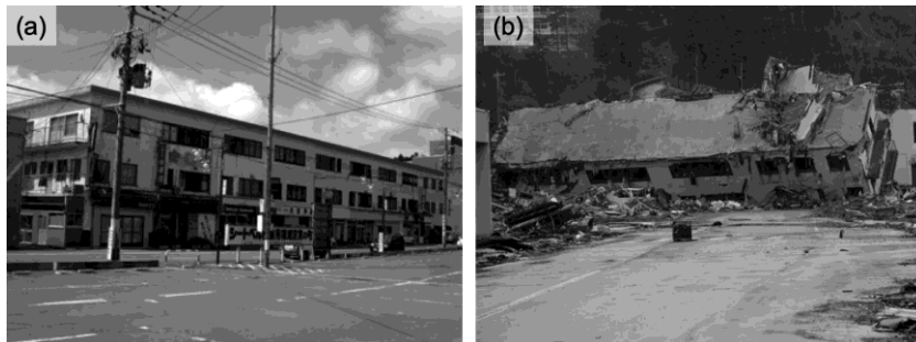
Fig.5. Photos of Building D taken before and after tsunami (Photo (a) [15])
